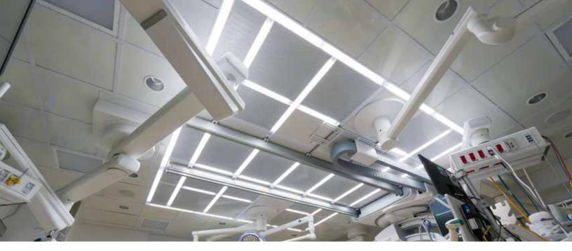
All elements are prefabricated and delivered to the construction site ready for assembly. Modular construction allows for our ceiling system to adapt to the needs of each room and specialization. FreedomAire is made of environmentally friendly materials, and the panels are designed for high mechanical strength and corrosion resistance. FreedomAire is easy to clean, resilient in extreme temperatures, and aesthetically pleasing. Skytron takes a consultative approach to building your OR.
